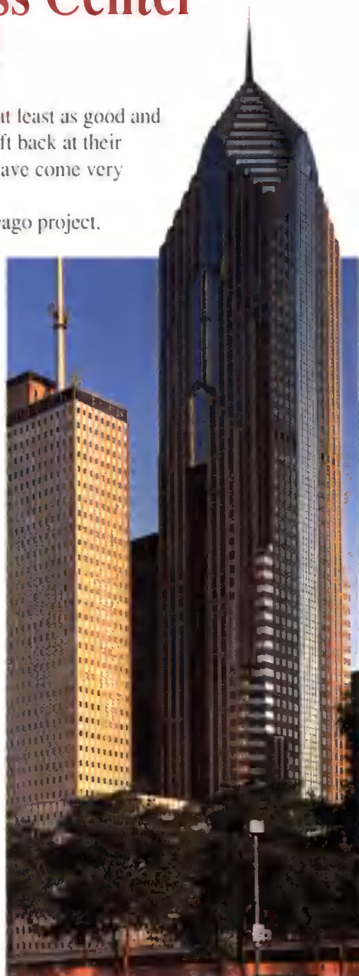
TAI-Chicago is on the 44th floor of Two Prudential Plaza, one of the world's great office centers.
