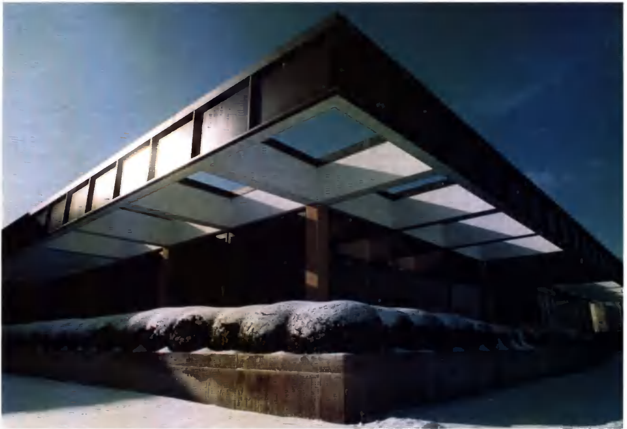
With the installation of the voice response system, Detroit Edison's Customer Communications Center (above) can handle 42,000 calls per hour.
